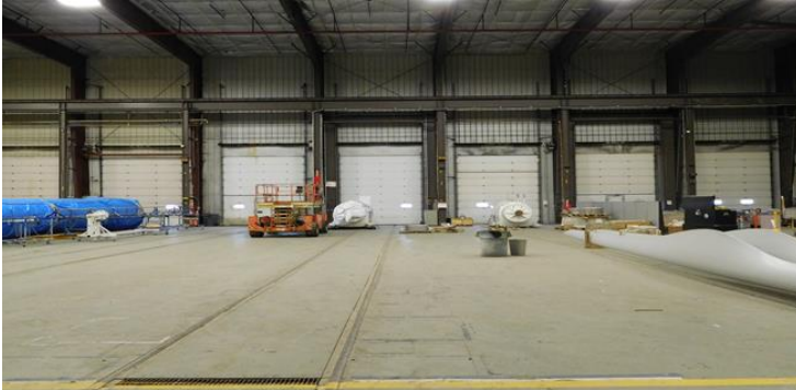
Internal High Bay
